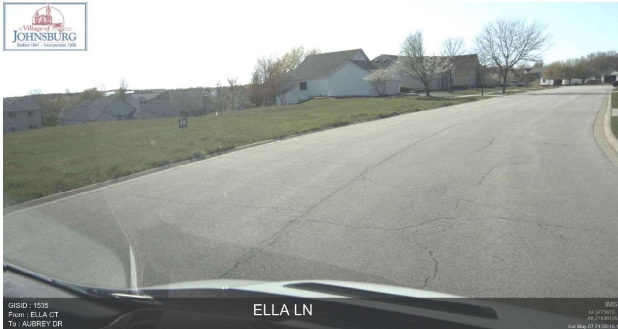
Figure 12 - Example of a Pavement Rated as Fair
