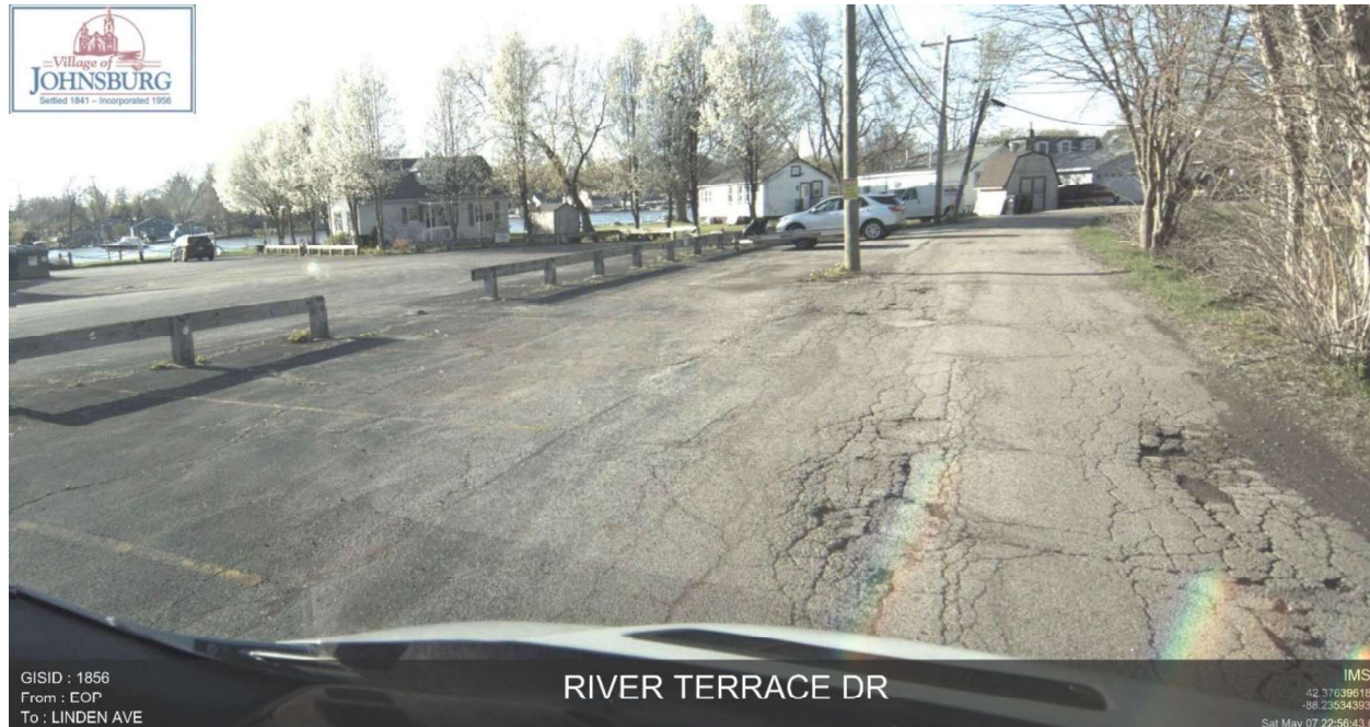
Figure 8 – Example of a Pavement Rated as Failed
