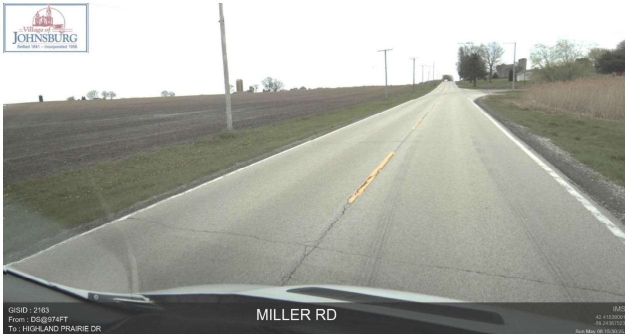
Figure 13 - Example of a Pavement Rated as Satisfactory
